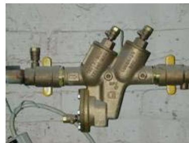
It is used for services that have either health hazards or non-health hazards and under conditions of backpressure or backsiphonage. It provides the highest level of protection among the mechanical backflow prevention devices.
